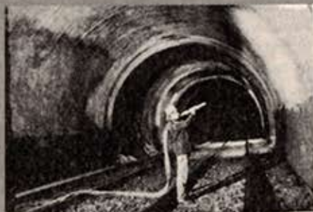
▲ Steel fibre shotcreting used for a tunnel lining job
