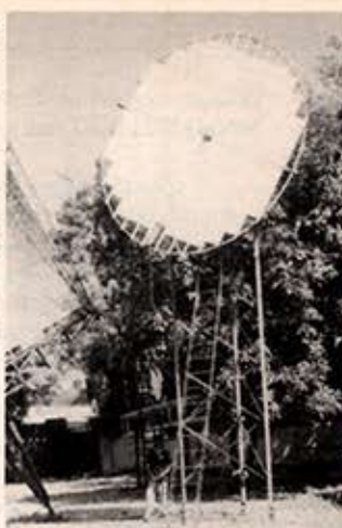
A solar concentrator erected at Baroda
