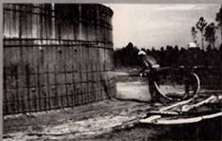
▲ Steel fibre shotcreting used for the construction of a large capacity ground level water tank.
