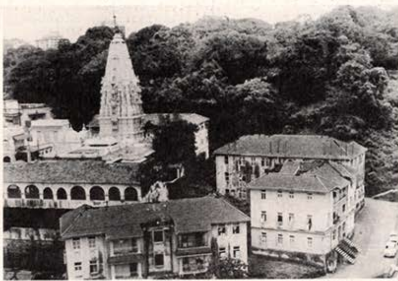
Parsi Fever Hospital (building on the left with arches) at the Muncherji Khareghat Colony
