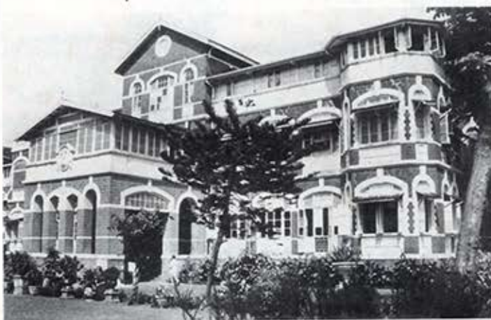
B. D. Petit Parsee General Hospital: under renovation
