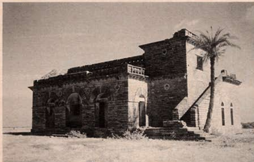
Bungli near the dokhma needs extensive repairs
