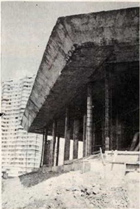
The agiary under construction at Godrej Baug
