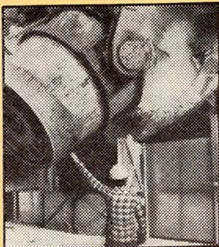
TISCO modernisation: Charging hot metal into the 130-ton LD converter
