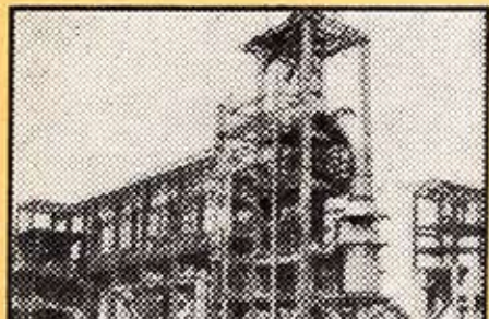
Sponge Iron Plant, Paloncha: DR unit with waste gas cleaning facility
