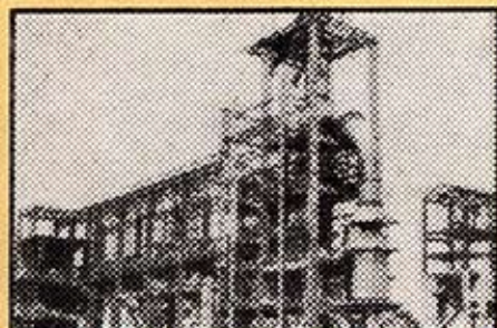
Sponge Iron Plant, Paloncha: DR unit with waste gas cleaning facility
