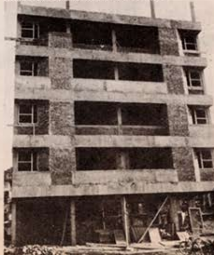
Construction in progress on the Divecha Trust land in Thana
