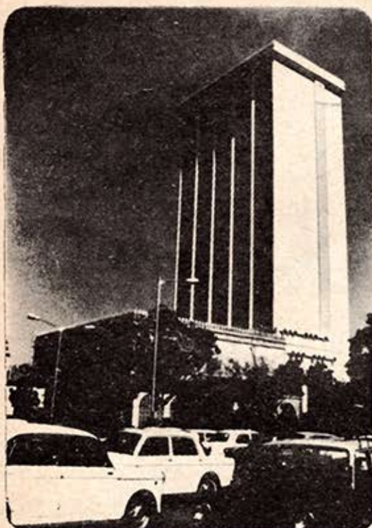
BAITUL HAJJAJ' BUILDING AT PALTON ROAD FOR THE HAJ COMMITTEE
