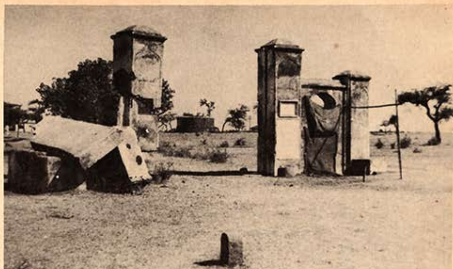
Two pillars minus gate and walls stand at the entrance to this dokhma on the outskirts of Surat.
