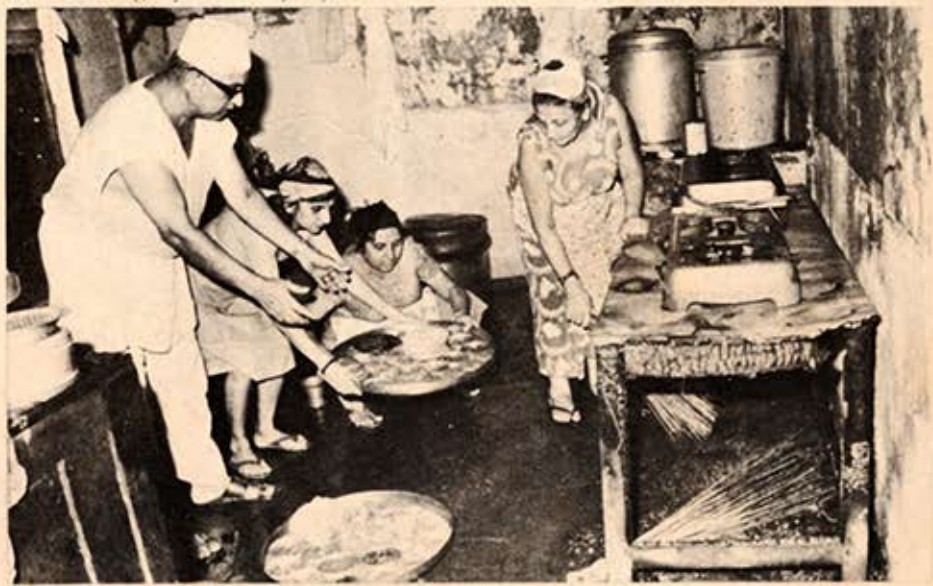
Ashberna Agiary kitchen after fire (Photo: Rashid Bamanbehram)
