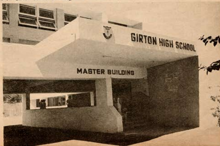
New Girton School building on Sleater Road.
