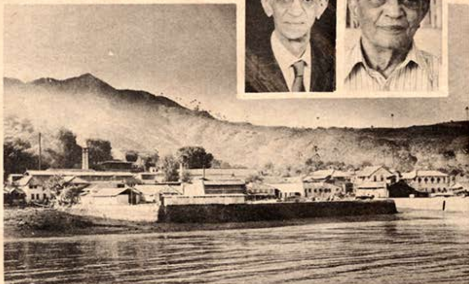
Old Bharat Tiles factory in Uran, (inset) Pherozesha and Rustom Sidhwa (right)
