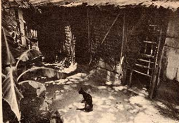
Left: The dilapidated shack which houses three families
