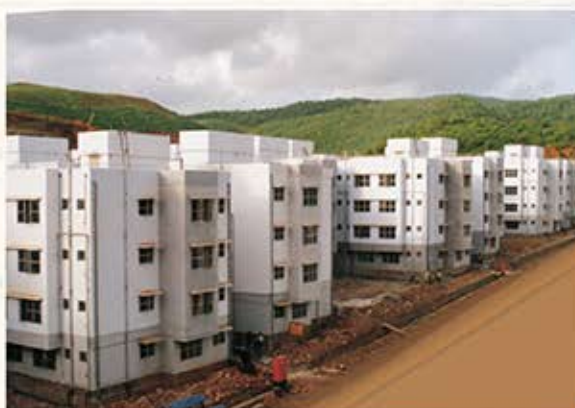
Petit Tower (left) and mass housing for the Nagari Nivara Parishad
