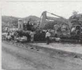
Mumbai - Pune Express Way
