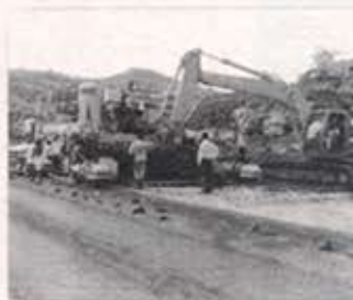
Mumbai - Pune Express Way
