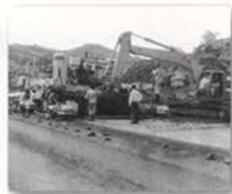
Mumbai - Pune Express Way
