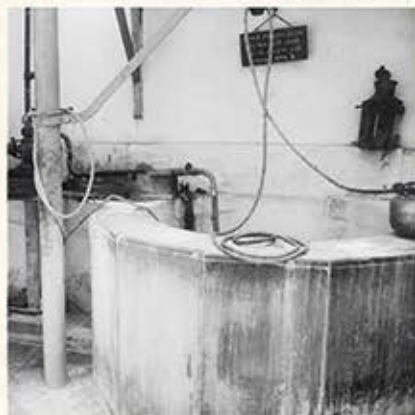
An agiary well serving as a reservoir of underground water
