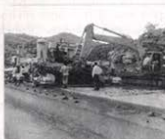
Mumbai - Pune Express Way
