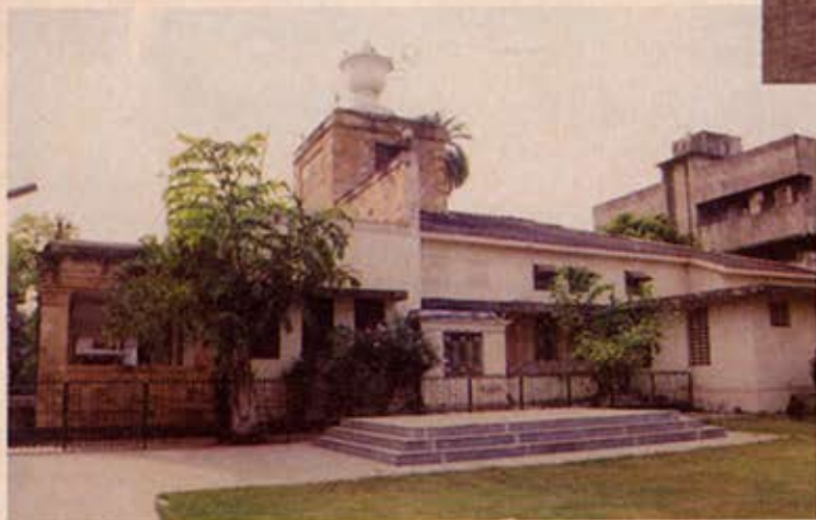
Clockwise from top: the Dharamshala facade; Gandhi Sagar Lake across the road; Mullan Dar-e-Meher adjacent to the Dharamshala and one of the rooms
