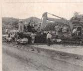
Mumbai - Pune Express Way
