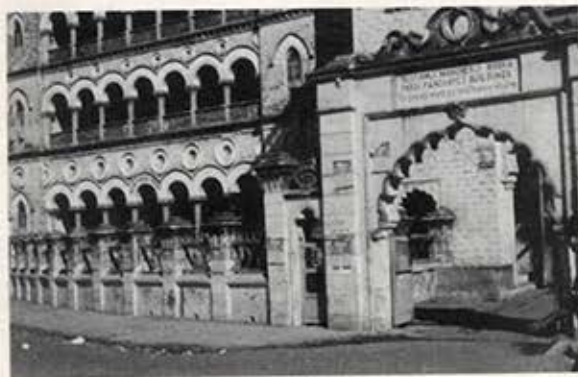
Headquarters of the Surat Parsi Panchayat
