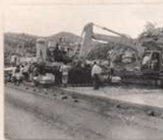
Mumbai - Pune Express Way
