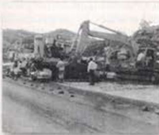
Mumbai - Pune Express Way
