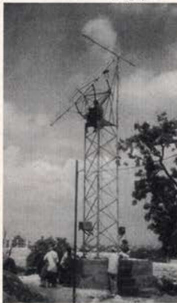
Solar concentrator installed at Secunderabad
