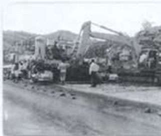
Mumbai - Pune Express Way
